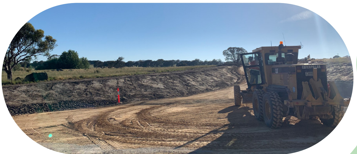
Photo: Site entry works at Rye Park Wind Farm, NSW
