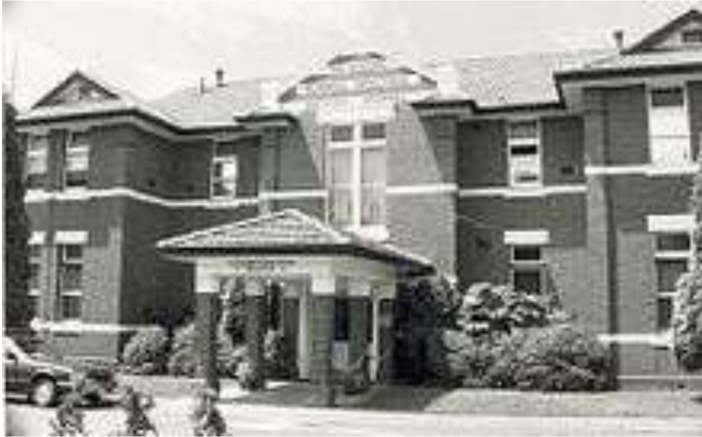
Fairfield Hospital, Victoria
